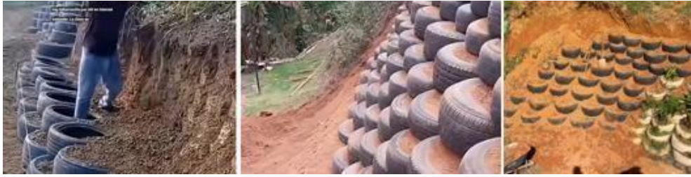
Figure 3 - Graphic representation of walls with tires. Own photograph, 2025.
