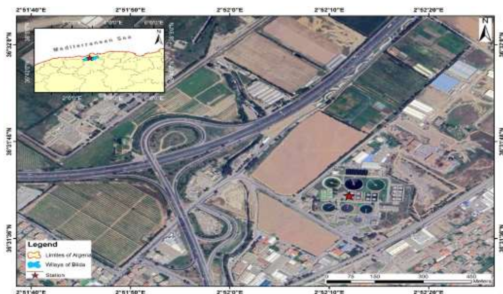
Figure 1. Aerial view of the Beni Merrad wastewater treatment plant (Blida, Algeria), showing the wastewater and sludge treatment units (Original, 2025).
