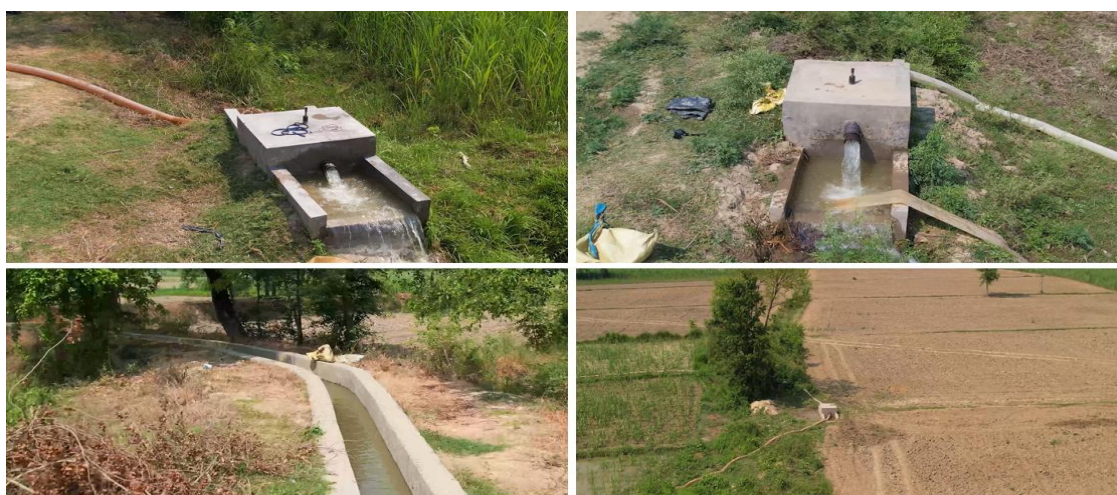
Figure 7. Irrigation Water Distribution in the Hriday Nagar Command Area
